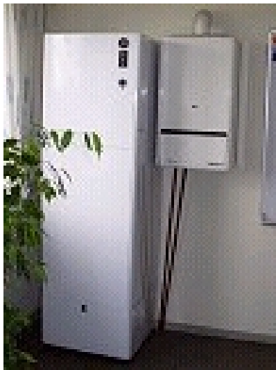
Figure Fejl! Ukendt argument for parameter. Solar storage (202 litres) from Batec together with gas boiler
