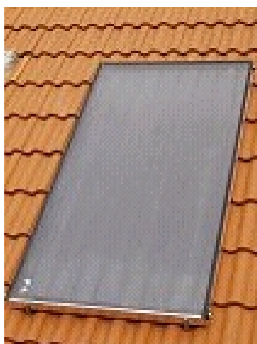
Figure Fejl! Ukendt argument for parameter. Flat plate single glazed solar collector panel from Batec
